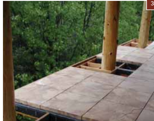
1 Frame deck with 4" joists 23 7/8" on center
